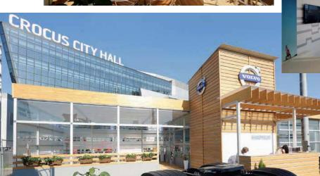
with its approx. 600 m² presence. The design was based on SYMA-MOL-TO90 combined with decorative larch elements, coordinated to VOLVO's corporate design and worldwide standards. The robust connectors and outstanding stability of SYMA-MOLTO made it possible to realise the 250 m² glass-walled pavilion in the terrace and air-conditioned lounge area to a depth of 6 metres without trusses.
